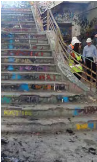
FIGURE 52 - INTERNAL STAIRCASE WITHIN SOUTH FREMANTLE POWER STATION
