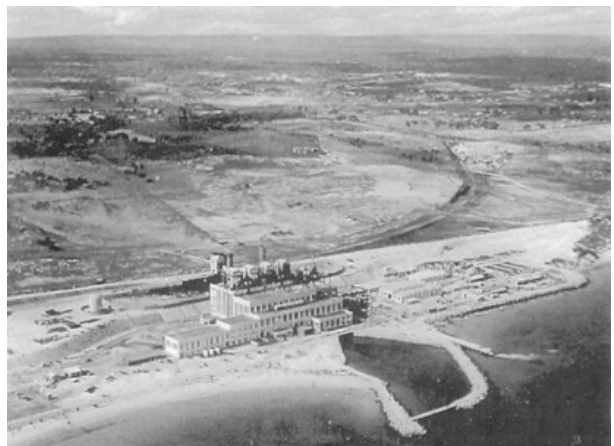
FIGURE 31 - SOUTH FREMANTLE POWER STATION (1953) SOURCE: EDMONDS, L; CATHEDRALS OF POWER PG 38
