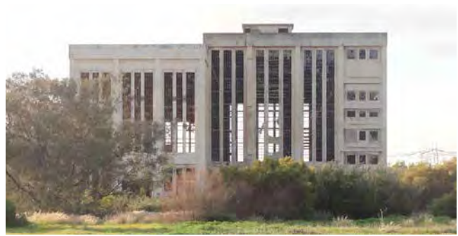
FIGURE 46 - SOUTH FREMANTLE POWER STATION
