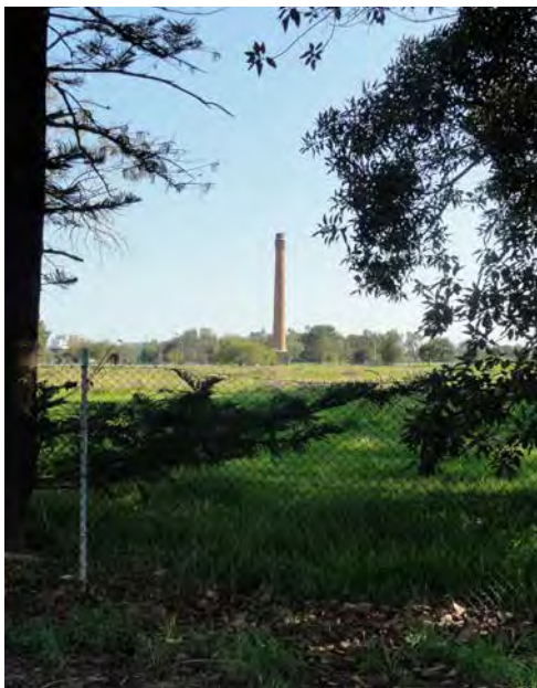
FIGURE 71 - ROBB JETTY CHIMNEY
