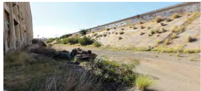
FIGURE 48 - SOUTH FREMANTLE POWER STATION AND COAL STORE
