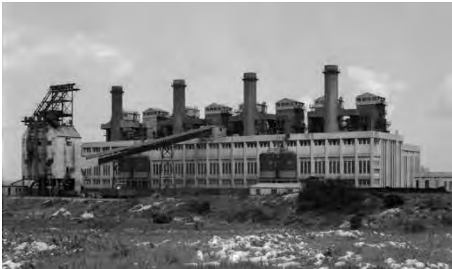
FIGURE 12 - SOUTH FREMANTLE POWER STATION (1957) SOURCE BATTYE LIBRARY 239097PD
