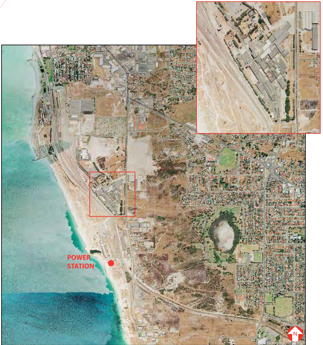
FIGURE 18 - AERIAL 1995 - INSET SHOWING THE EXTENSIVE OPERATIONS OF THE ROBB JETTY ABATTOIR, WHICH WAS DEMOLISHED IN 1995
