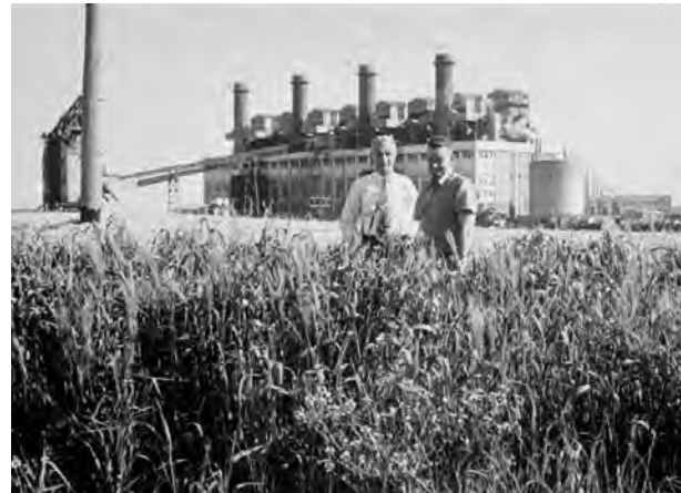
FIGURE 30 - SOUTH FREMANTLE POWER STATION (c1964) SOURCE: FREMANTLE CITY LIBRARY LOCAL HISTORY COLLECTION IMAGE NUMEBR 2497
