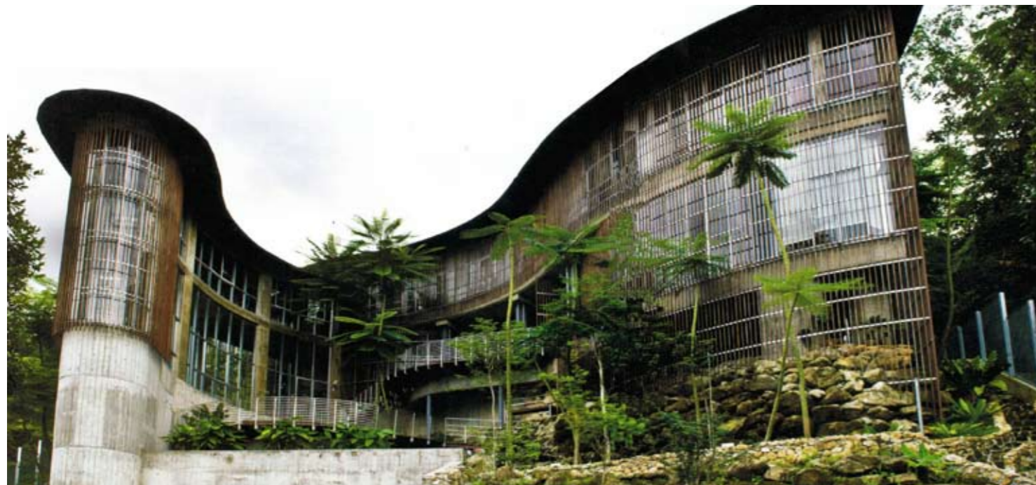
ABOVE: The reference image above is indicative of the type of atmosphere that could be achieved in the Emplacement precinct through the integration of landscape, vegetation and natural materials that have the potential to create a new topography in built form enhances the existing landscape.
