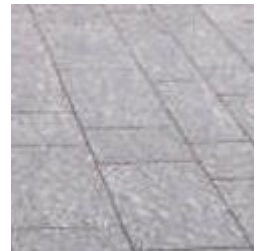
shared path & median_ milled concrete pavers
