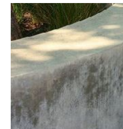
wall material_ formed concrete walls
