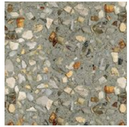
shared path_ washed aggregate concrete
