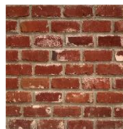
wall material_ recycled brick walls
