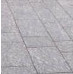
shared path & median_ milled concrete pavers
