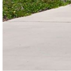
shared path_ brushed concrete
