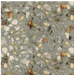
shared path_ washed aggregate concrete
