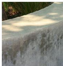
wall material_ formed concrete walls
