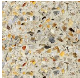
shared path_ washed aggregate concrete
