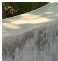
wall material_ formed concrete walls
