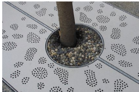
typical custom tree grates with specific patterning depending on precinct and theming area
