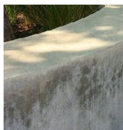
wall material_ formed concrete walls
