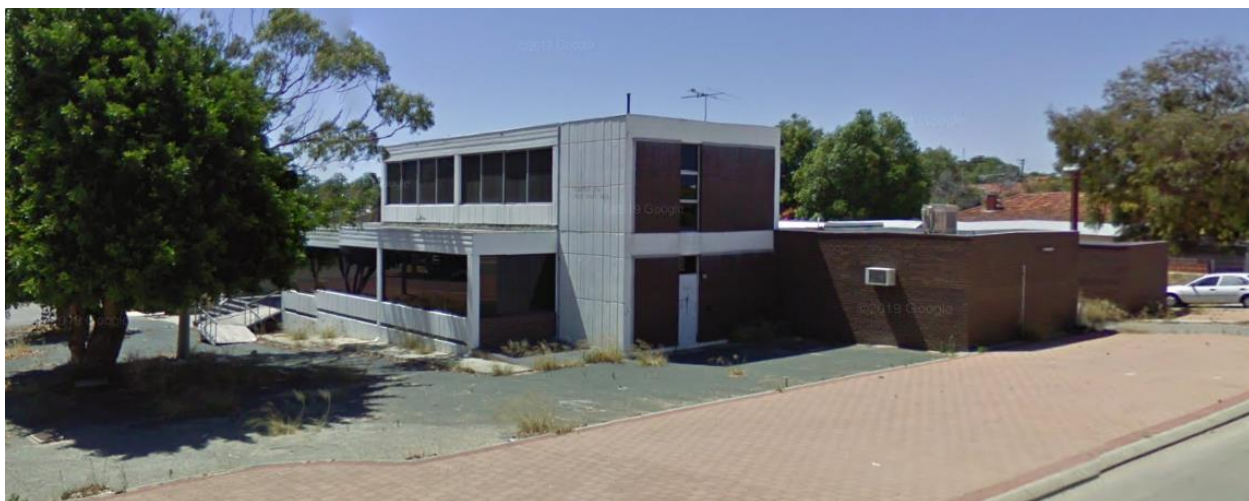
Figure 4. View of former post office from Straughair Street
