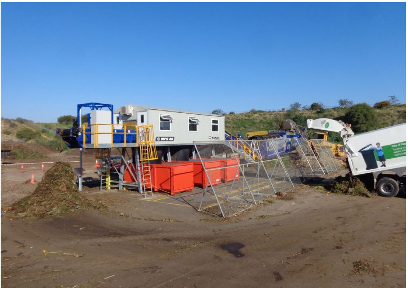
City of Cockburn garden organics sorting facility at Henderson Waste Recovery Park.
