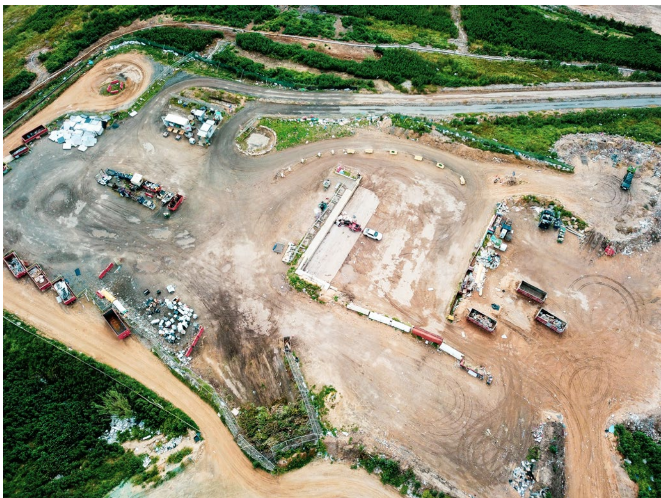
Aerial image of the Henderson Waste Recovery Park Transfer Station.
