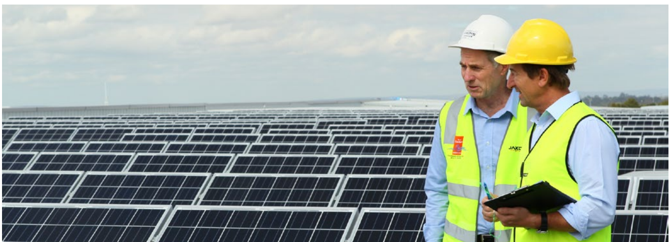
Solar photovoltaic system (130kW), Cockburn Health and Community Facility.
