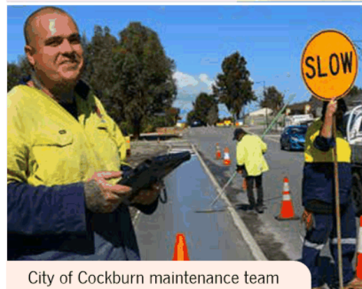
Hammond Road upgrade
