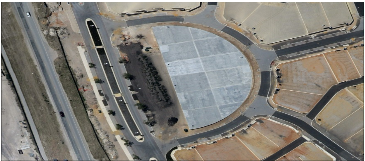
Figure 4.2.1 8500m 3 capacity network storage tank at Lucretia Park, January 2008
