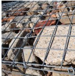
wall material_ gabion walls
