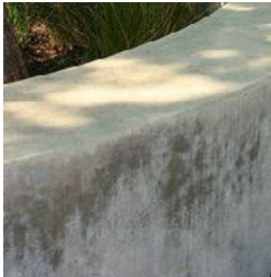
wall material_ formed concrete walls
