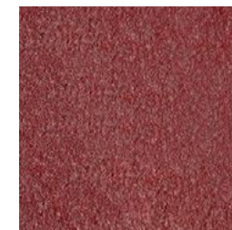
parking bays_ red asphalt
