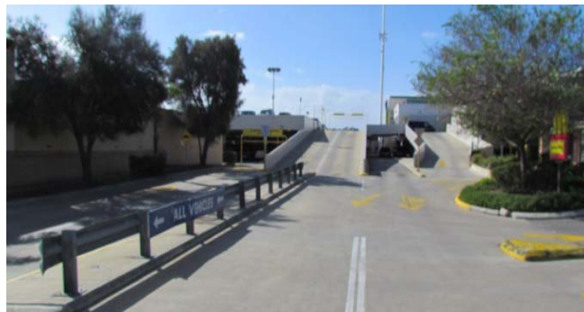
Figure 14. Ramp from Rockingham Road
