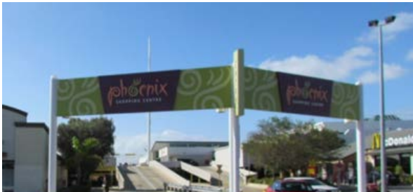
Figure 17. Rockingham Road vehicle entrance to upper deck parking - relies on signage
