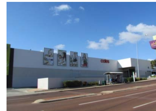
Figure 20. Rockingham Road servicing area
