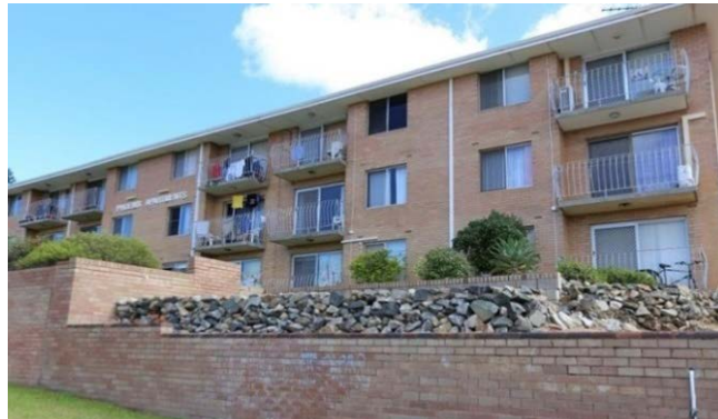
Figure 22. Glendower Way, Spearwood – 24 single bedroom apartments
