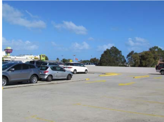
Figure 36. Existing expansive upper deck car parking
