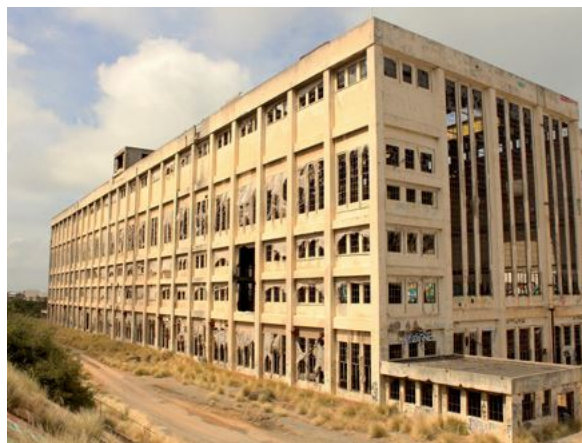
power station precinct_vibe image
